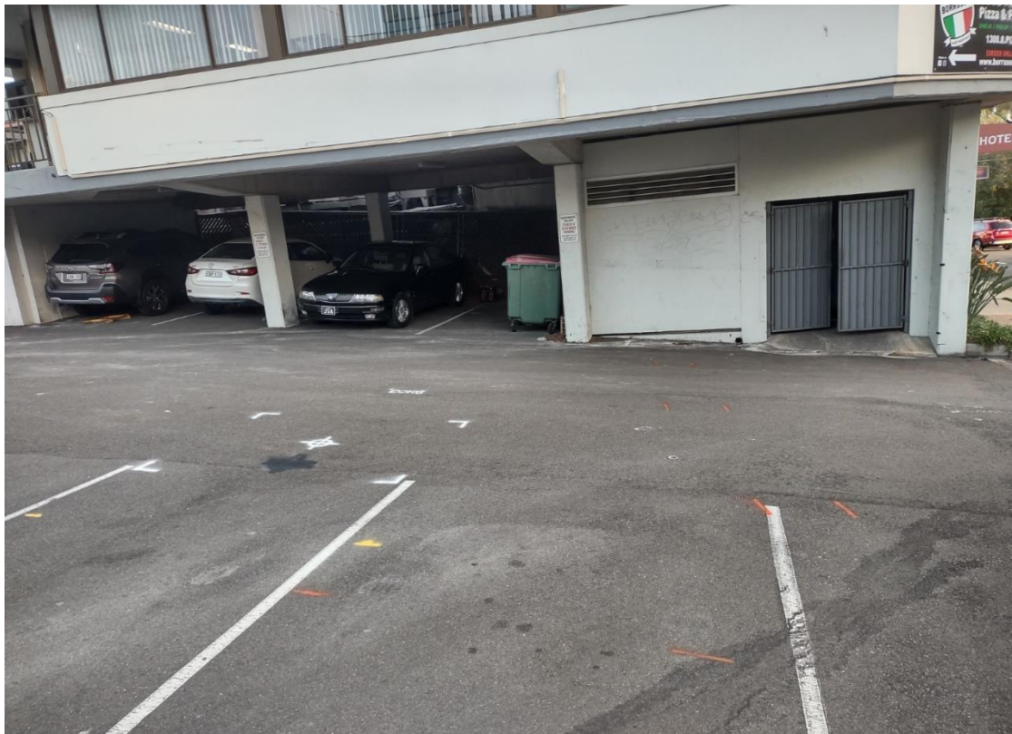
Photo 2: General site condition, car park, facing south
