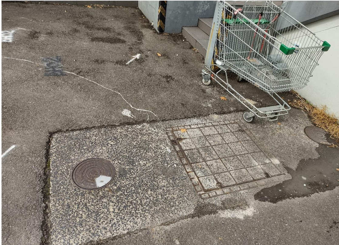
Photo 3: Car park area, grease trap
